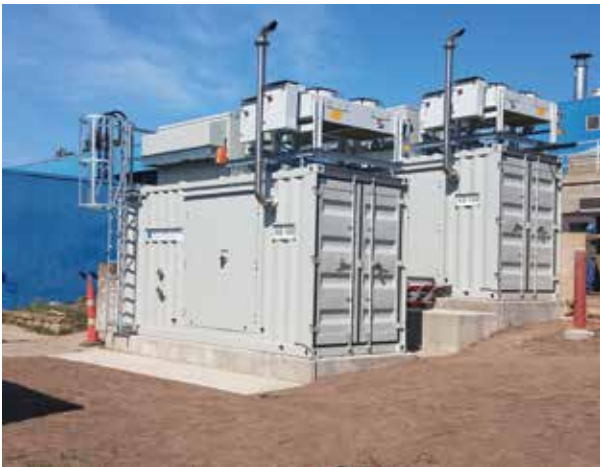
Twin KB 100 Biogas CHP Modules Pictured above
