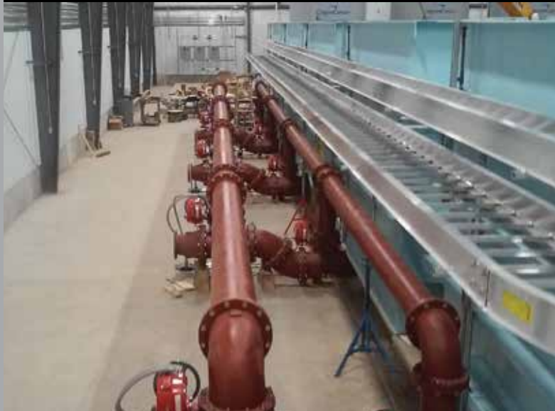
Interim Facility Pipe Manifold and Tanks Center Township
