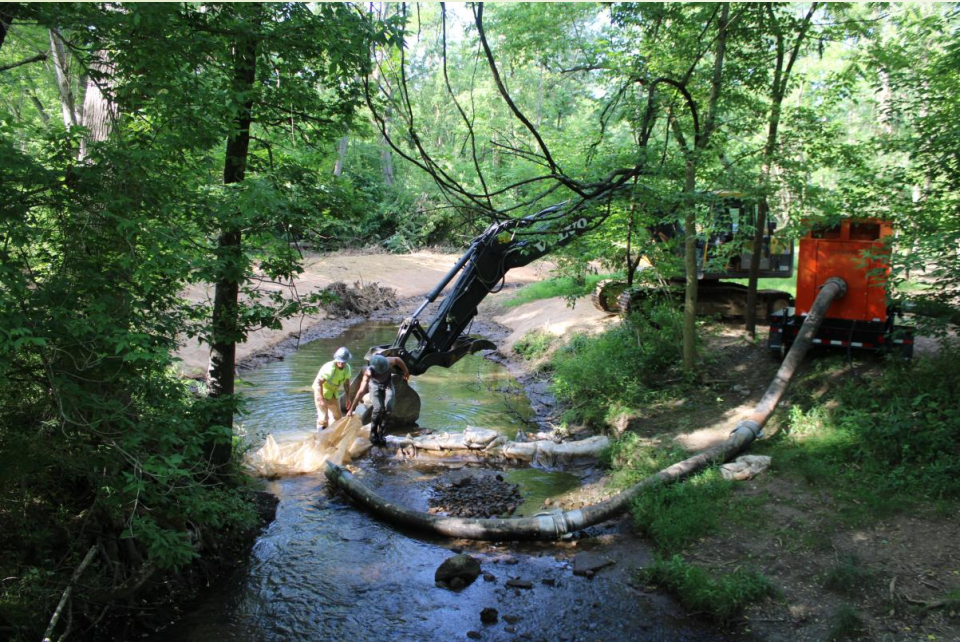
Newly graded banks with erosion blanket
