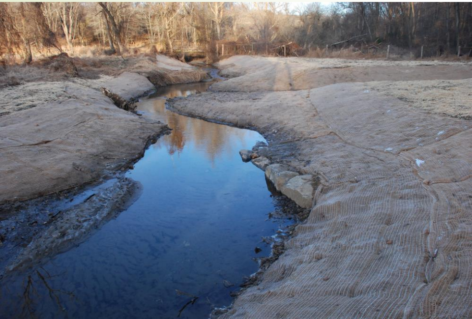
Newly graded banks with erosion blanket
