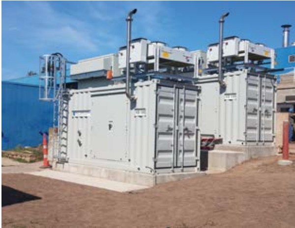
Twin KB 100 Biogas CHP Modules Pictured above
