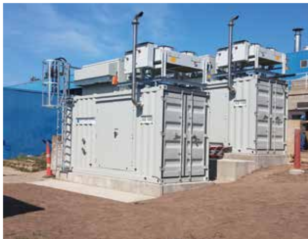
Twin KB 100 Biogas CHP Modules Pictured above
