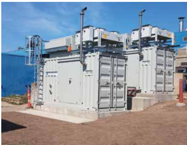
Twin KB 100 Biogas CHP Modules Pictured above
